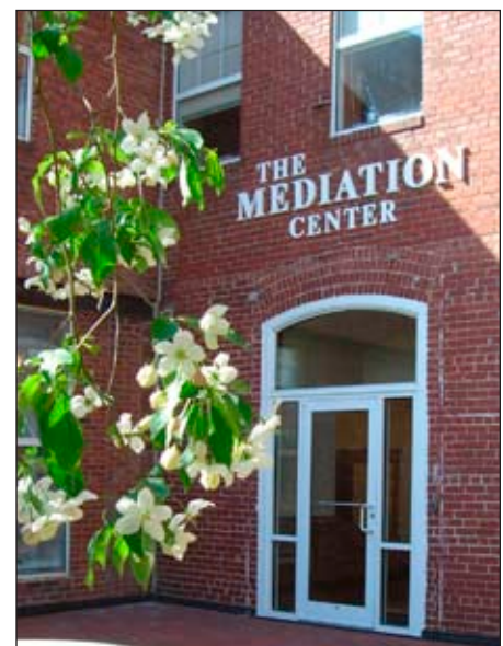
New front entrance of The Mediation Center, Lincoln.
